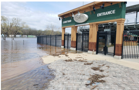
Flooding at Copeland Park on April 23 (credit: NWS La Crosse)
