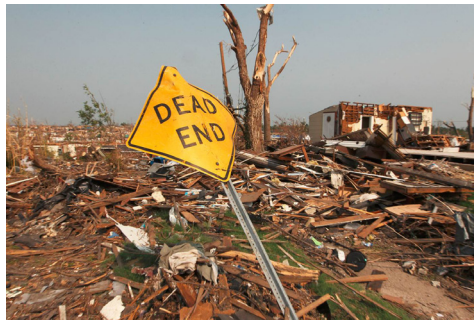
Complete destruction of a neighborhood in Joplin, MO following an EF-5 tornado on May 22. (Source: KMOV News 4, St. Louis)
